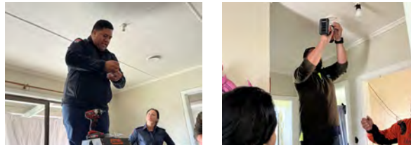
Ngā Kaimahi Taiwhenua installing new smoke alarms
